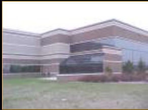
Building Finished Exterior
